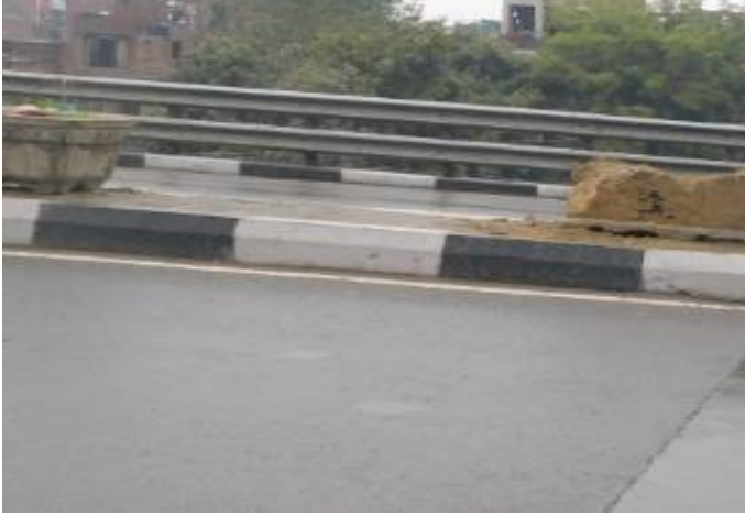
Photo 43. Kerb Stones in the median
