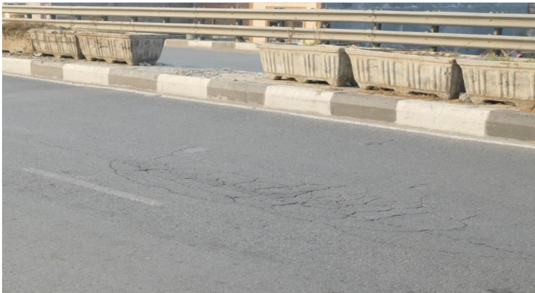
Photo 49. Distressed pattern on wearing coat
