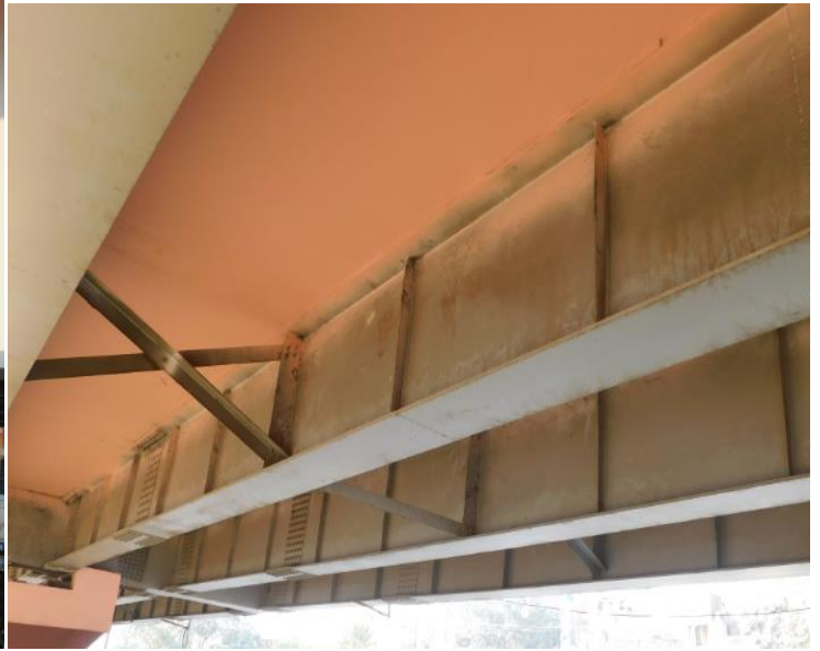
Photo 21.a) Inner Steel girders with cross bracings
