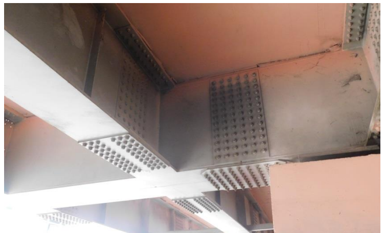
Photo 23.a) End Diaphragms with no distress
