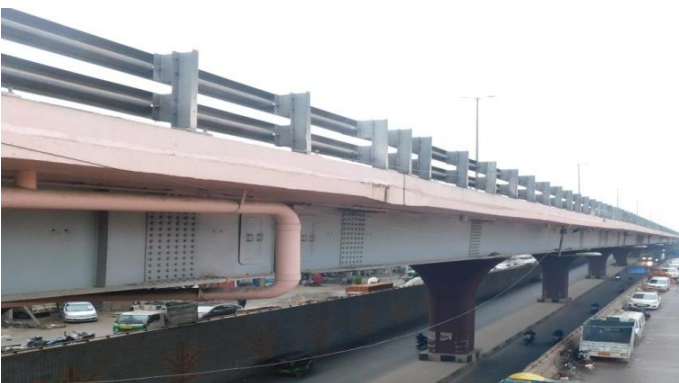
Photo 47. Outlet pipes are not connected to the downtakes
