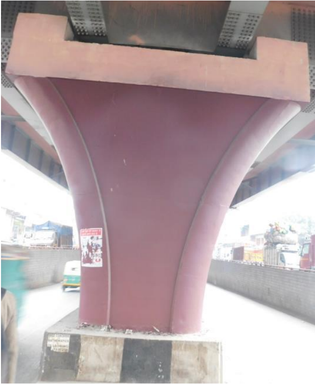
Photo 35. Piers showing no distress or damages
