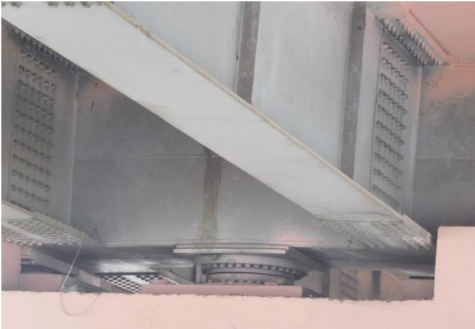
Photo 24. Steel girders connection with bearings
