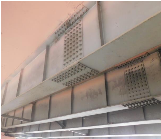
Photo 22. Steel girders showing no sign of corrosion
