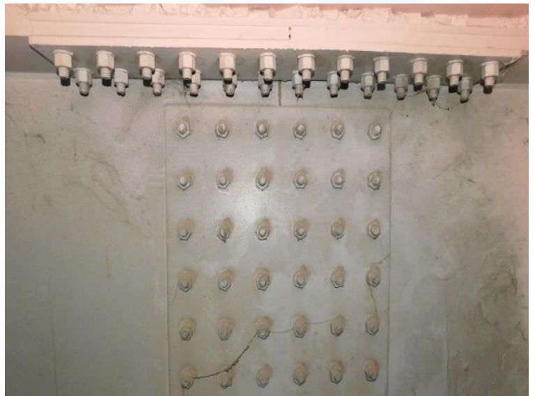
Photo 22.a) Steel bolt connection
