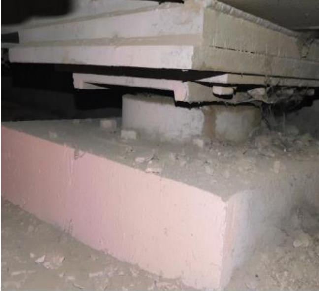
Photo 39. Bearings without any damages
