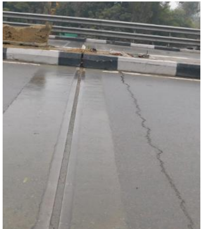
Photo 34. Transverse crack due to tension near Expansion joints
