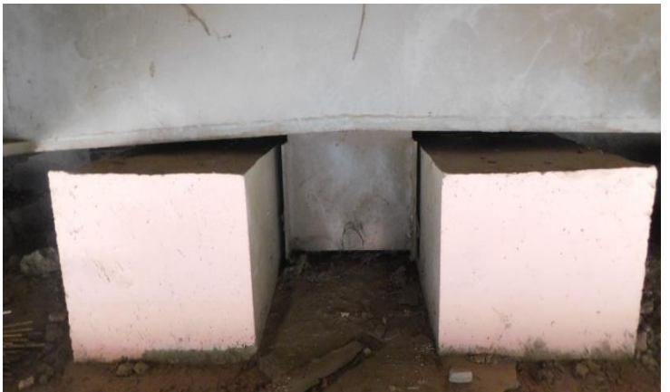
Photo 42. Seismic Restrainers showing no distress or damage
