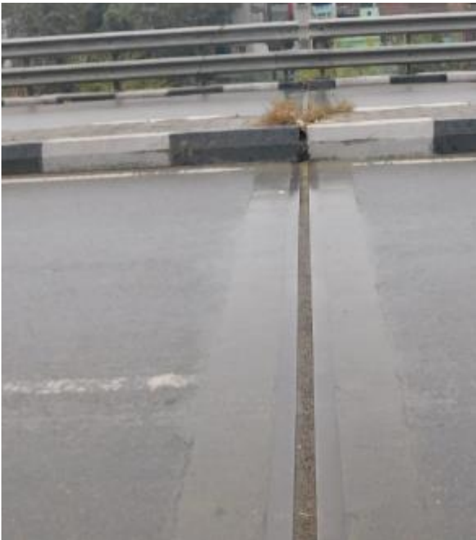
Photo 33. No damages in expansion joints
