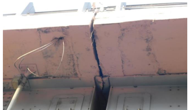
Photo 47.a) Drainage pipe missing.
