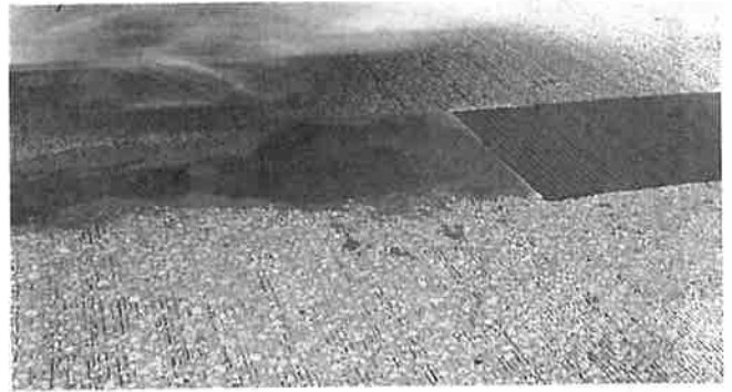
FIGURE 5 Spalls patched with asphalt and walking spalls.
