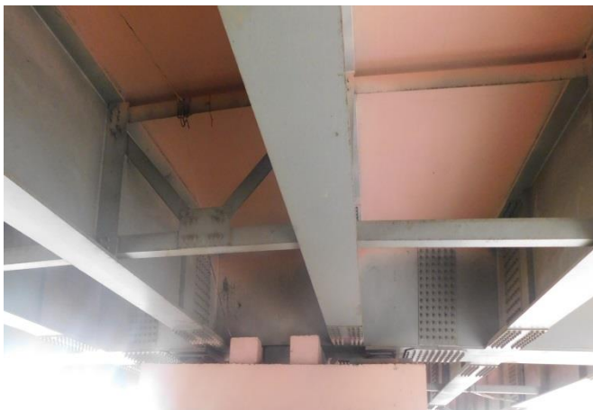
Photo 23. Cross and rectangular bracings
