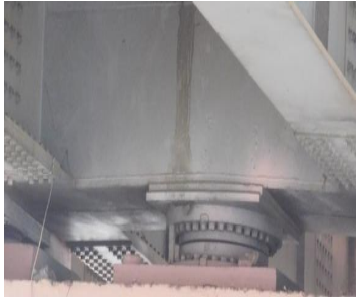
Photo 40. Bearings are in good condition
