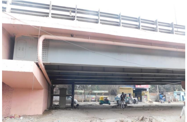
Photo 24.a) Girders resting in abutments
